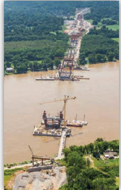
Walsh-Vinci on the East End Bridge project.
