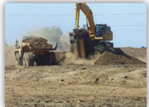
Fisher Contracting moving dirt at Toyota in Georgetown, Kentucky
