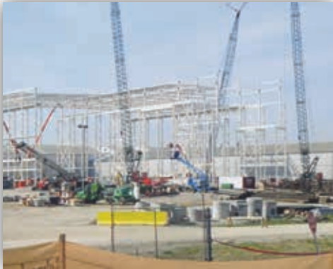
Midwest Steel at the Aleris expansion in Hancock Co. Kentucky
