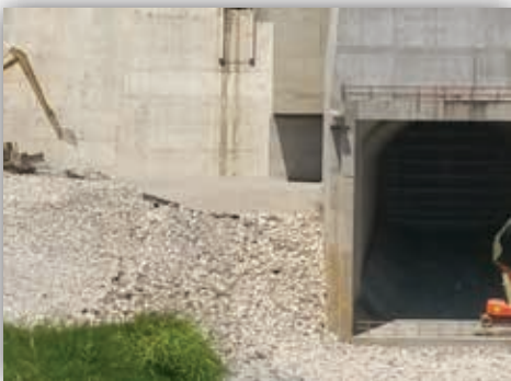
Morsey Constructors and Barnard Construction at the Smithland Hydro Dam.
